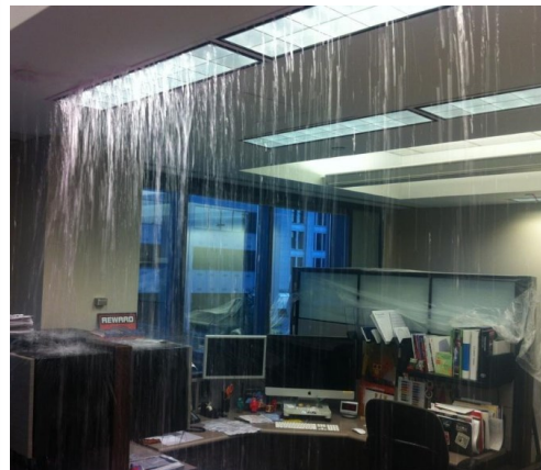
Figure 1: Water can cause costly damage to computer equipment.
